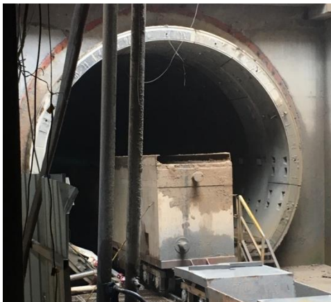
Figure 9. The entrance of one of the tunnels. The large cart is used to remove the soft sediments and transport them to the surface by crane.
